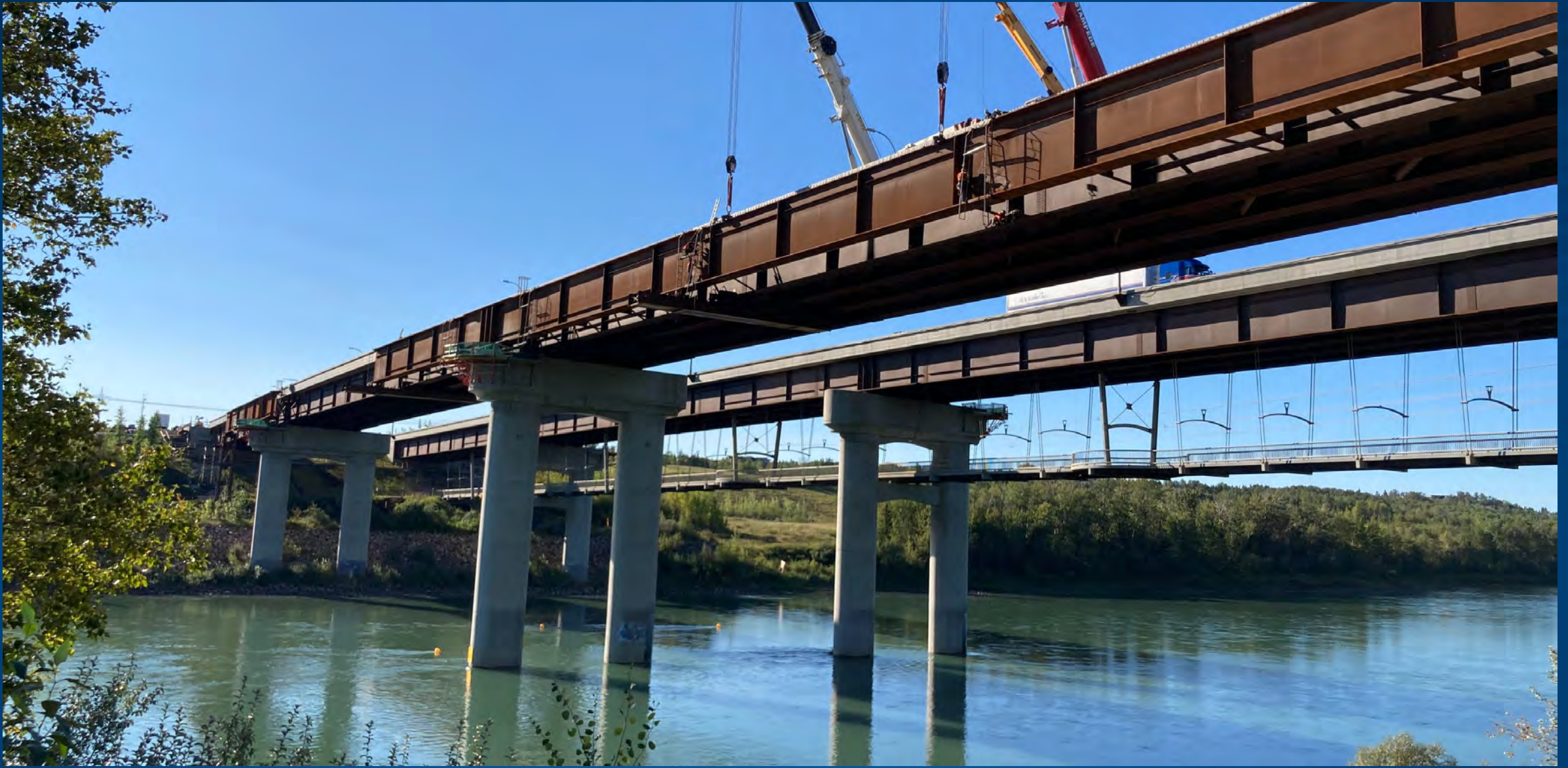
SWAHD over the North Saskatchewan River - Construction
