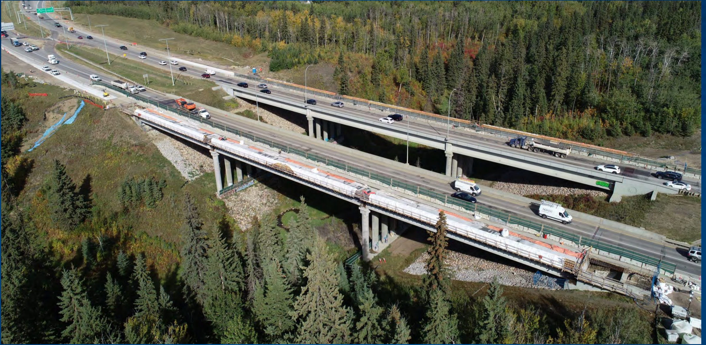
SWAHD over Wedgewood Creek - Construction
